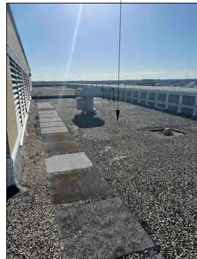
NORTH SIDE OF MAIN ROOF, SOUTH SIDE ROOF OPPOSITE HAND
