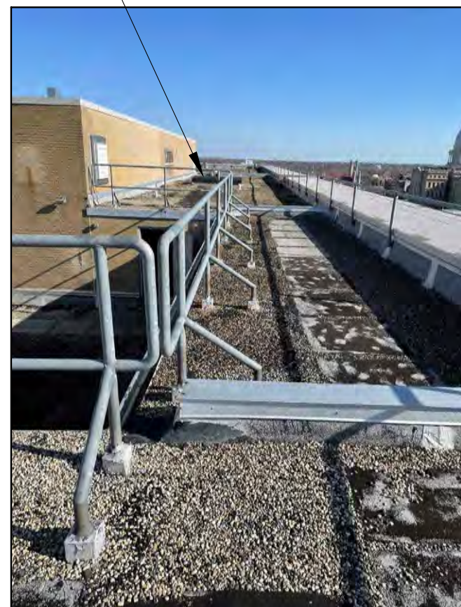
RAISE CURB OF EXISTING MECHANICAL ROOM ACCESS DOOR HATCH TO ACCOMMODATE NEW INSULATION THICKNESS FOR PROPER FLASHING DETAIL
