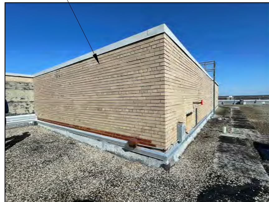
RAISE CURB OF EXISTING MECHANICAL ROOM ACCESS DOOR HATCH TO ACCOMMODATE NEW INSULATION THICKNESS FOR PROPER FLASHING DETAIL
