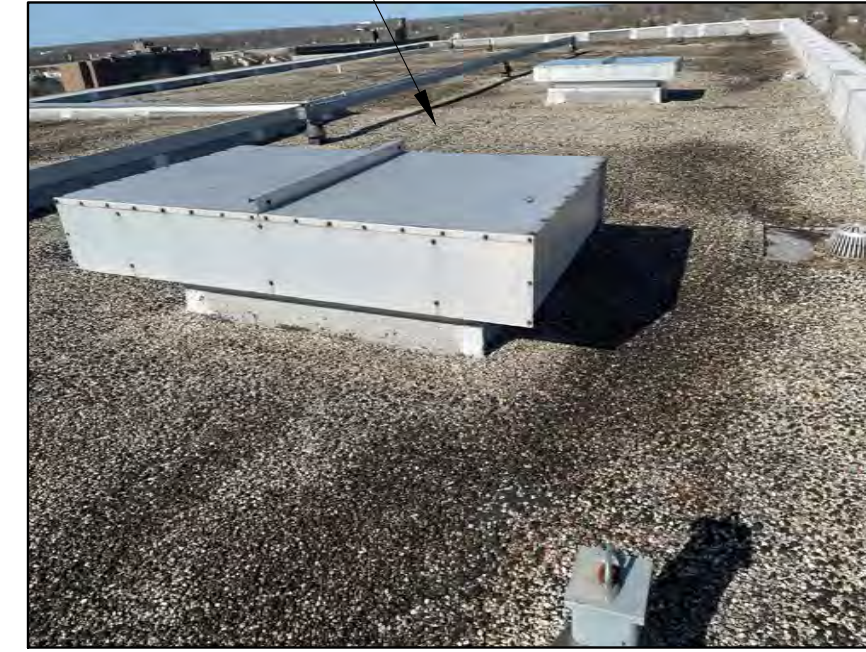
RECESSED ROOF AREA: LOWEST SECTION. NEW EPDM TO EXTEND FULL HEIGHT OF BRICK WALLS TO MAIN ROOF EDGE. REPLACE GUTTER AND DOWNSPOUTS.
