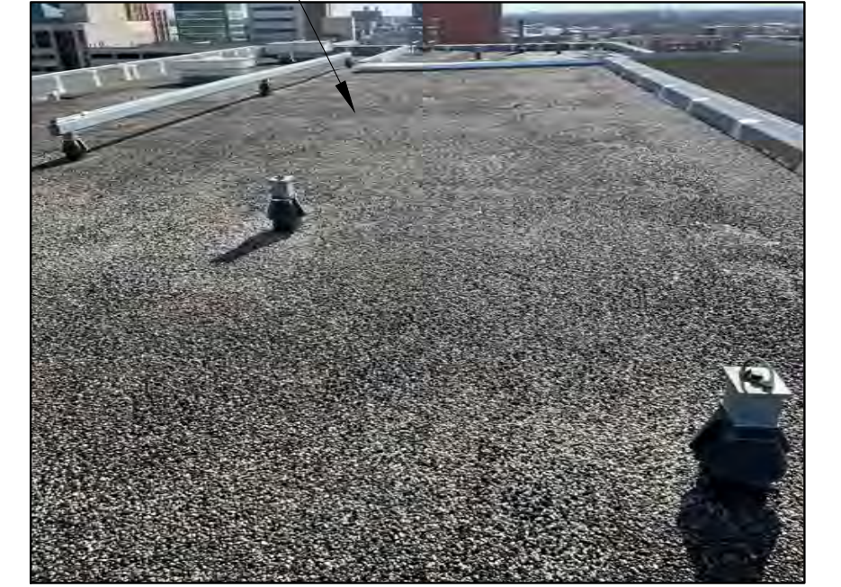
RECESSED ROOF AREA: LOWEST SECTION. NEW EPDM TO EXTEND FULL HEIGHT OF BRICK WALLS TO MAIN ROOF EDGE. REPLACE GUTTER AND DOWNSPOUTS.
